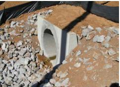
Specified in the plans or special provisions. Use straight headwall only in locations where pipe exposed end does not face the direction of traffic.
