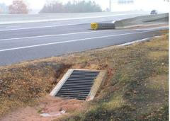
Use **Pipe End Structure** (719-615-00) when specified in the plans or special provisions. Use pipe end structure in locations where pipe exposed end faces the direction of traffic. Pipe end structures may be used in other locations if approved by the RCE.
