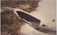
Use **Beveling of Pipe End** (719-610-00) when specified in the plans or special provisions. Beveled ends may only be used on flexible pipe up to 24" diameter and on rigid pipe up to 60" diameter. When beveling of pipe ends is specified on flexible pipe larger than 24" diameter, install pipe straight headwall, pipe end structure, flared end section, or wingwall section. Use factory fabricated beveled ends for all pipe types unless approved by the Engineer.
