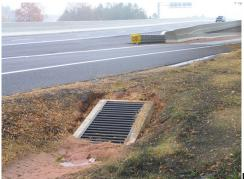
Use Pipe End Structure (719-615-00) when specified
