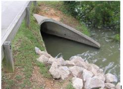
Use **Pipe Flared End Section** when specified in the plans or special provisions.
