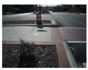
Pedestrian Refuge Island — Pedestrian element that provides resting space. Minimum length = 6'-0"; DWS required each side regardless if design is cut-through or uses curb ramps.
