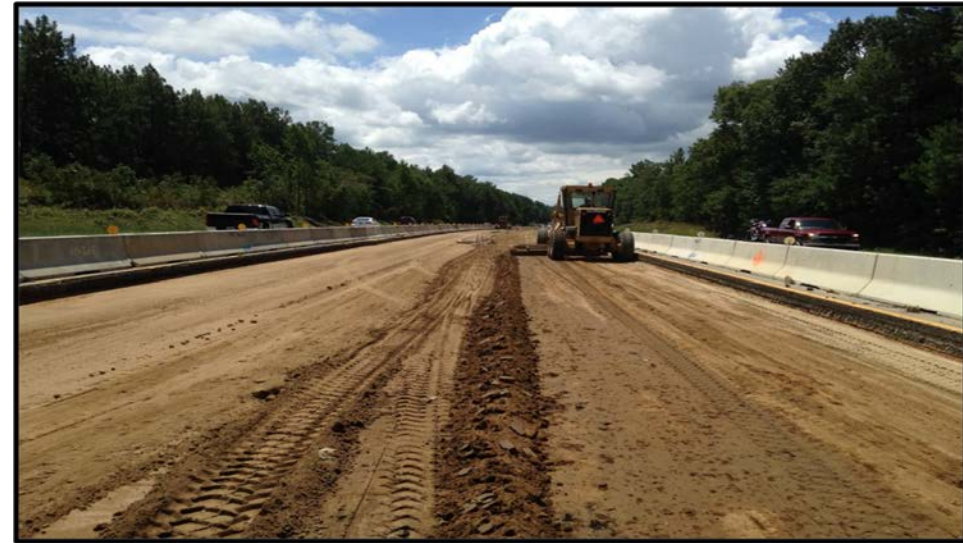
I-26 Widening & Rehab Lexington/Calhoun Counties
