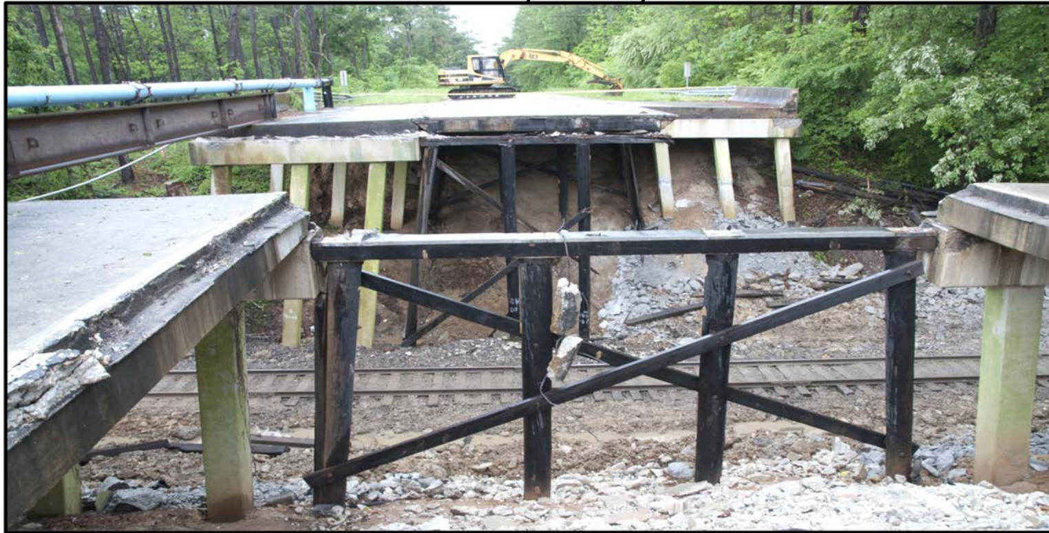
Cypress Gardens Emergency Bridge Berkeley County
