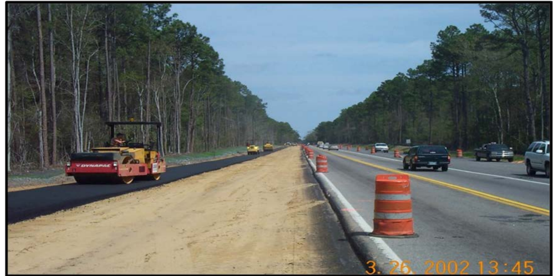
SC 170 Widening Beaufort County
