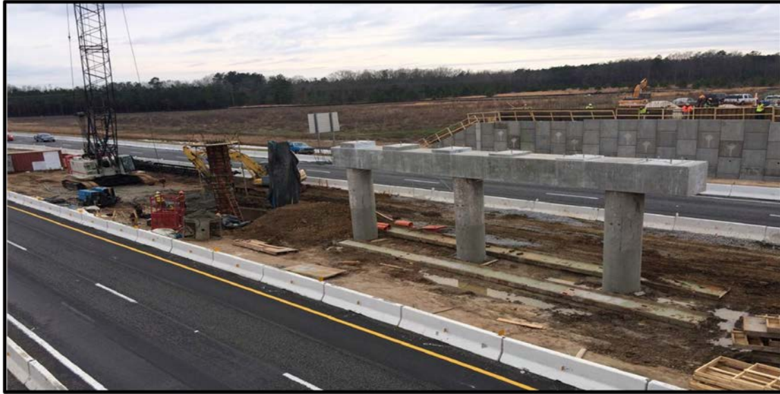
I-95/US 301 Interchange Orangeburg County
