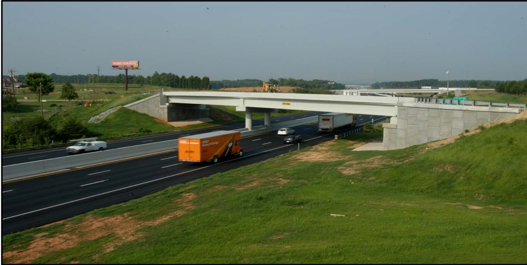
Brockman-McClimon Interchange (I-85 Access Improvements) Spartanburg County
