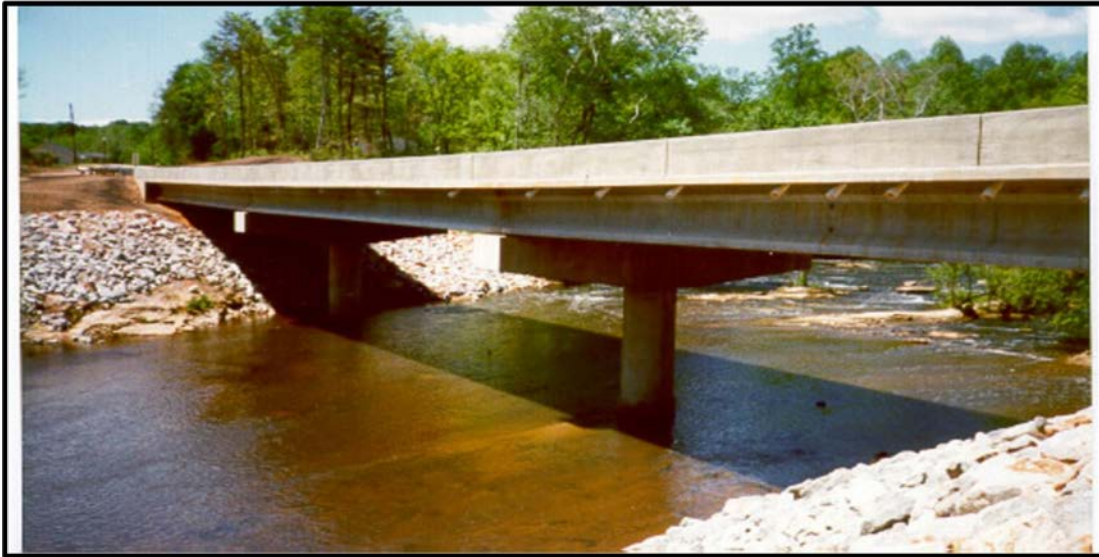
Reedy River Bridge Greenville County
