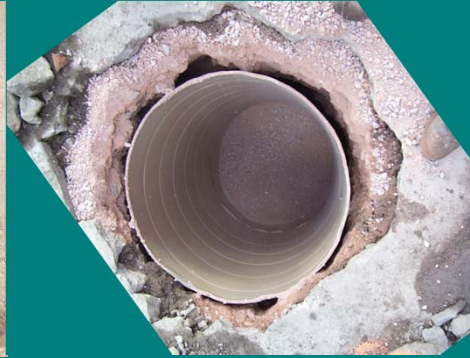
Redesign using 30" sonotube (longer, narrower footing)
