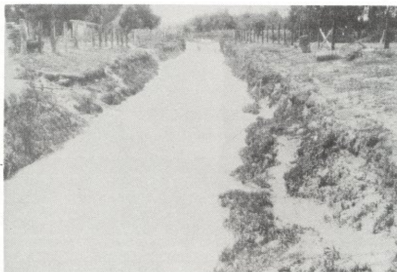
Cypress Creek Dredged Channel near Bethel Springs, Tennessee. Approximate bottom width 15 feet. Picture taken 1917.
