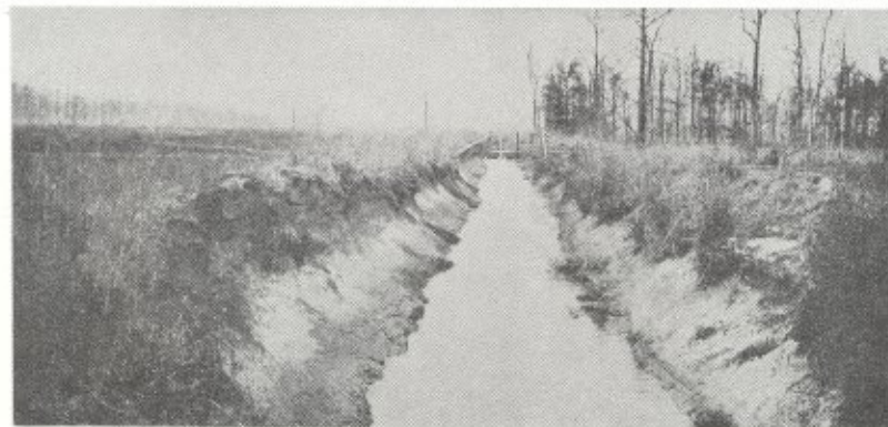
Chawappah Creek Dredged Channel near Shannon, Mississippi. Approximate bottom width 15 feet. Picture taken 1913.
