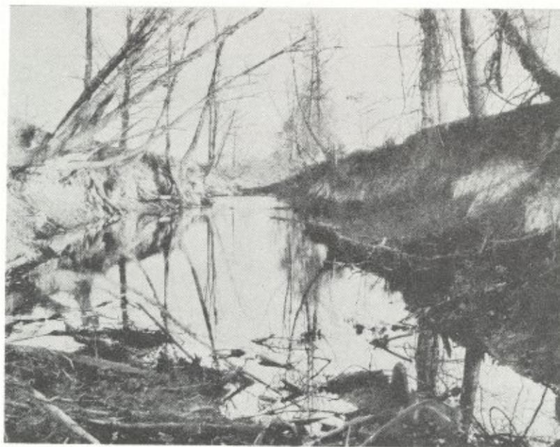
South Forked Deer River-Old Straight Channel-Jackson, Tennessee. Approximate bottom width 25 feet. Picture taken in 1916.
