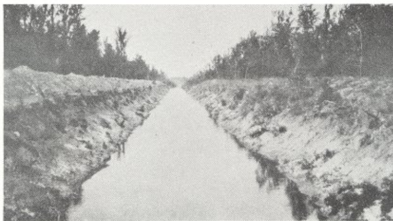
Bogue Phalia Dredged Channel near Helm, Mississippi. Approximate bottom width 45 feet. Picture taken in 1915.
