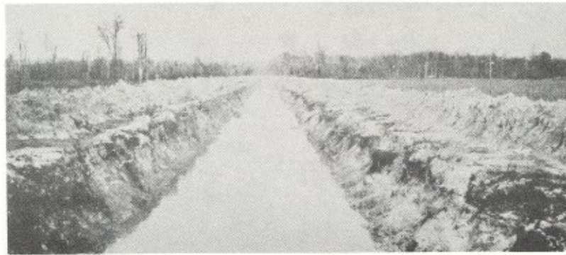
Mud Creek Dredged Channel near Tupelo, Mississippi. Approximate bottom width 10 feet. Picture taken 1913.
