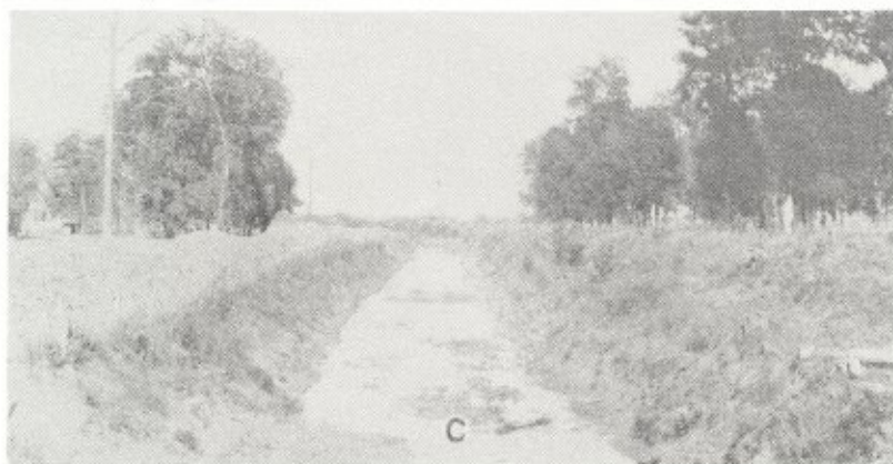
Horseshoe Bayou Dredged Channel near Cleveland, Mississippi. Approximate bottom width 25 feet. Picture taken May 1924.
