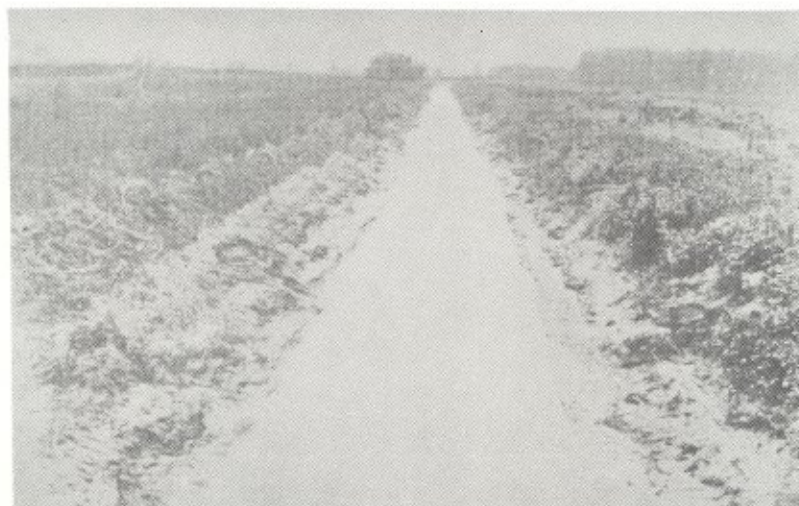
Pigeon Creek Dredged Channel near Cresent, Iowa. Approximate bottom width 15 feet. Picture taken in 1917.
