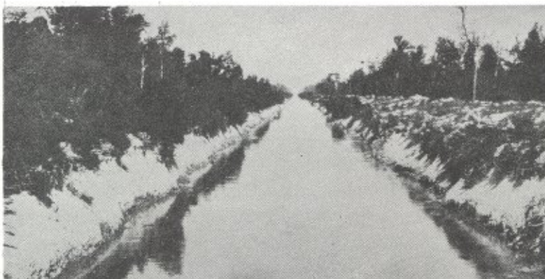
South Forked Deer River Dredged Channel near Roberts, Tennessee. Approximate bottom width 40 feet. Picture taken in 1916.
