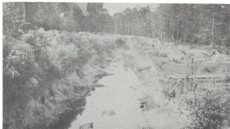
Sugar Creek Dredged Channel near Henderson, Tennessee. Approximate bottom width 15 feet. Picture taken 1917.
