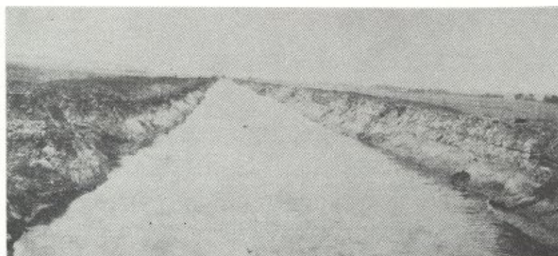
Boyer River Dredged Channel near Missouri Valley, Iowa. Approximate bottom width 40 feet. Picture taken in 1917.
