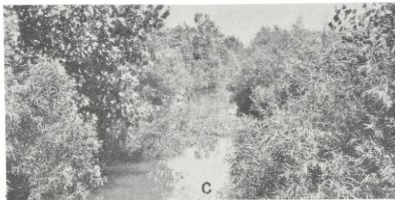
Camp Creek Dredged Channel near Seymore, Illinois. Approximate bottom width 15 feet. Picture taken July 1927.
