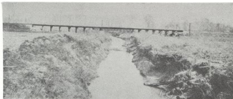
Coonewah Creek Dredged Channel near Shannon, Mississippi. Approximate bottom width 15 feet. Picture taken in 1913.
