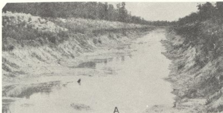
Dredged Ditch No. 43 of Cypress Creek Drainage District near Arkansas City, Arkansas. Approximate bottom width 55 feet. Picture taken July 1926.
