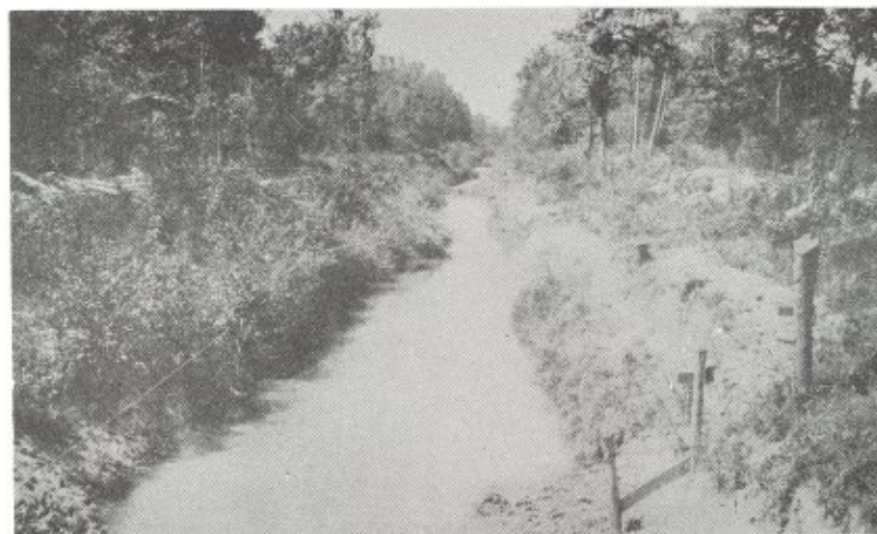
Huggins Creek Dredged Channel near Finger, Tennessee. Approximate bottom width 15 feet. Picture taken 1917.
