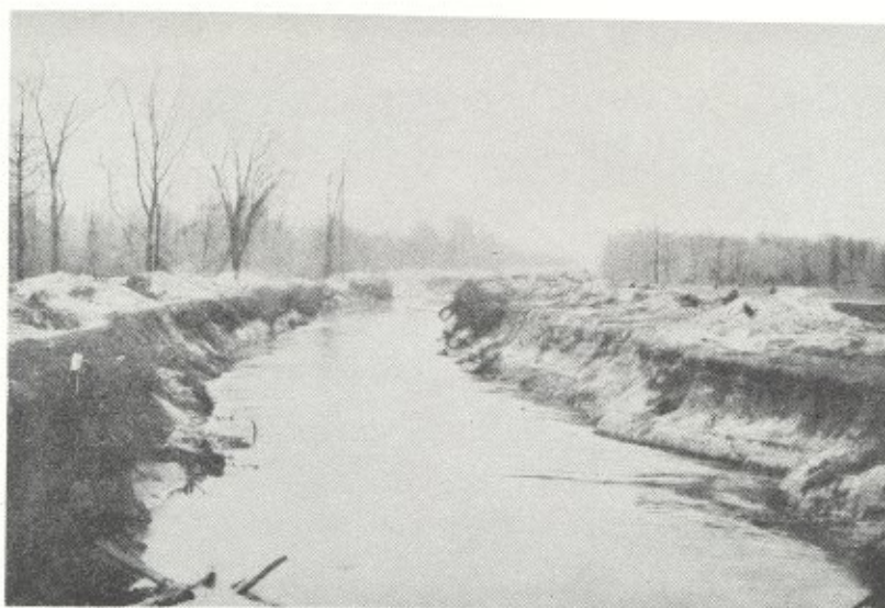
South Forked Deer River Dredged Channel at Cambells Levee - Jackson, Mississippi. Approximate bottom width 30 feet. Picture taken in 1916.
