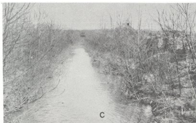
West Branch of Salt Fork Dredged Channel near Urbana, Illinois. Approximate bottom width 20 feet. Picture taken April 1925.
