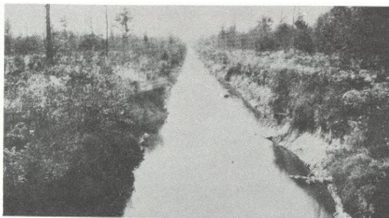
South Forked Deer River Dredged Channel near Henderson, Tennessee. Approximate bottom width 20 feet. Picture taken in 1916.
