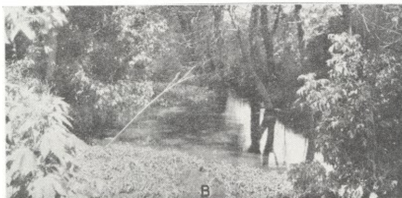
Kaskaskia Mutual Dredged Channel near Bondville, Illinois. Approximate bottom width 10 feet. Picture taken July 1927.
