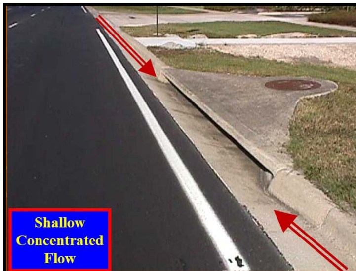
Figure 3.11. Shallow Concentrated Flow in a Roadway Gutter
