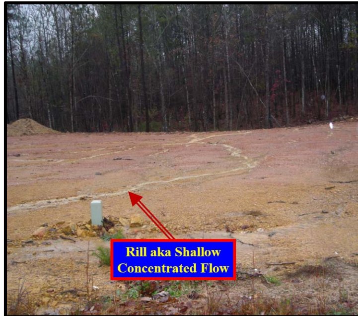
Figure 3.10. Shallow Concentrated Runoff from a Construction Site
