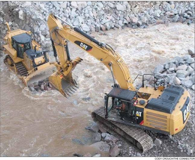
SCDOT closed the Jarvis Klapman Blvd. bridge over the Saluda River for work crews to dump large boulders into the Columbia Canal during the repair of the City of Columbia's water system.
