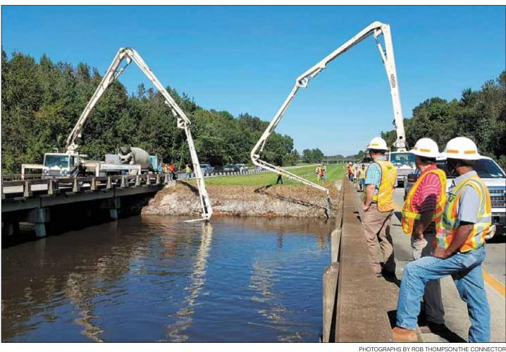
Scott McElveen, Michael Godwin and Wendell Jones of Clarendon Construction monitor concrete pouring underneath bridges along I-95 in Clarendon County on Sunday, Oct. 11. Six concrete pump trucks from United Contractors and SCDOT crews worked around the clock, seven days a week to shore up bridge pilings affected by flooding along the heavily traveled interstate.
