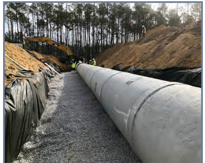
Installation of storm water pipe to improve drainage.
