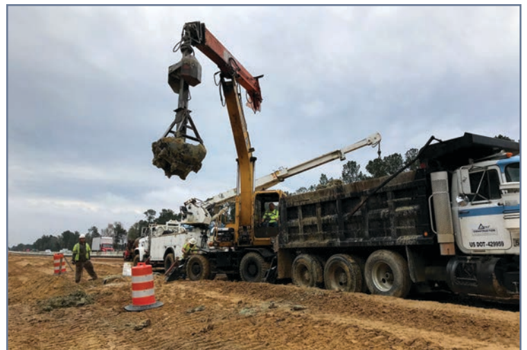
Installation of concrete foundations to support sign structures.
