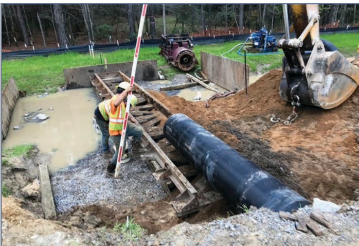
Volvo Interchange team working on drainage pipes.
