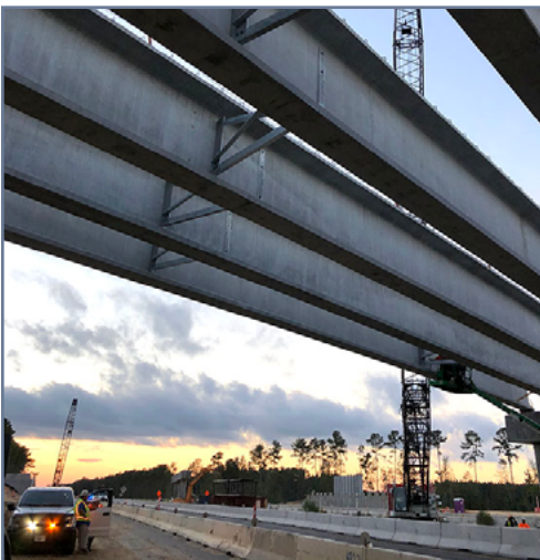
Bridge girders over I-26 Eastbound.
