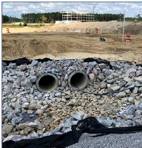
Drainage pipe installation.
