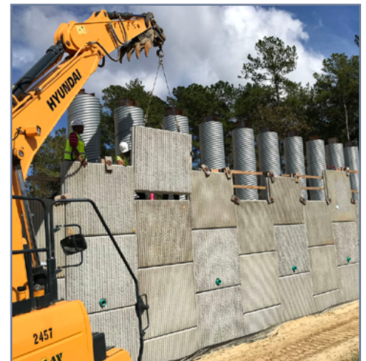
Wall and support structure construction for I-26 Westbound bridge girders.
