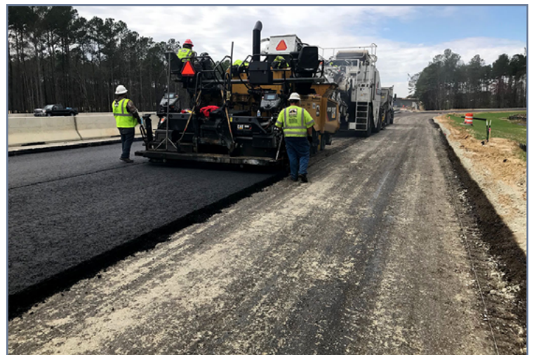
Asphalt pavement is underway along the Volvo Interchange ramps.
