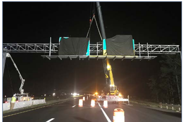
Overhead sign erection in progress.
