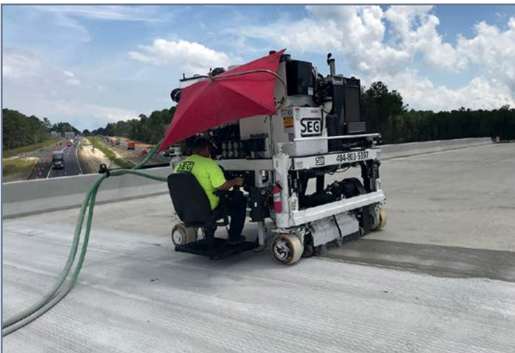
Grooving the bridge decks.
