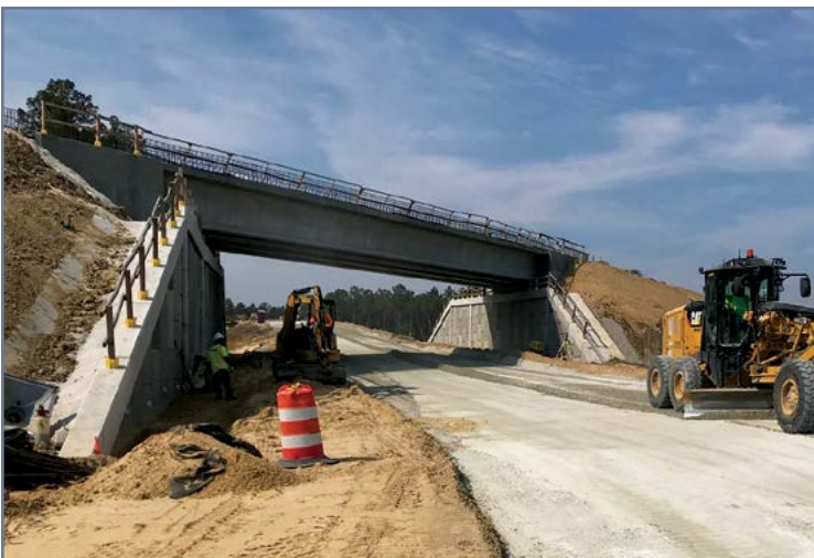
Preparation for asphalt paving.
