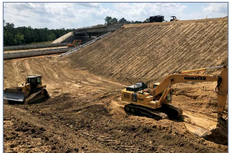
Major earthwork operations are complete.
