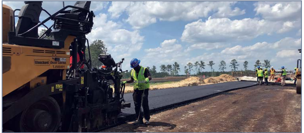
Asphalt placement continues to progress on the ramps.
